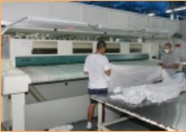
The new laundry at Changi Prisons Complex now offers greater capacity.
